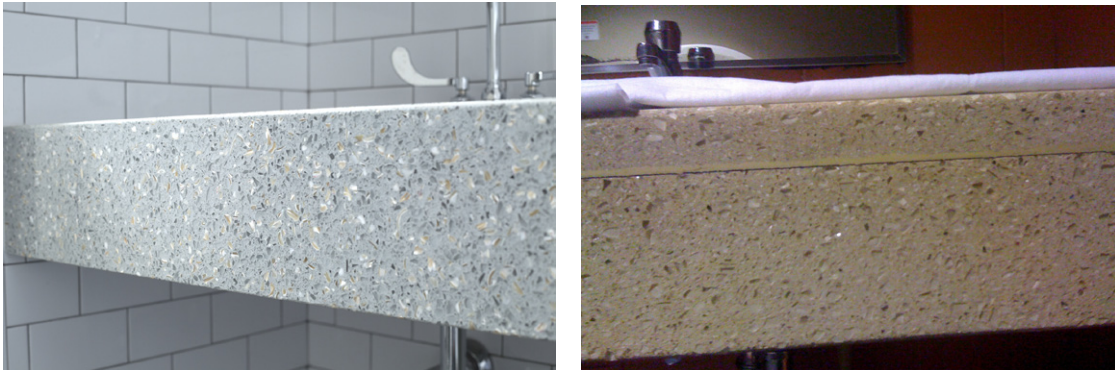
FIGURE 12 Example of properly built up edge (left), and improper stack lamination (right).
