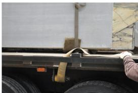
4. Add padding where the strap meets the slab at the top and at the bottom. The padding will reduce the tension on the slab during transit.
