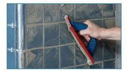
**Step 7** After a full 24 hours (some installations may require extended cure times) apply grout with a rubber grout float, forcing grout into joints until full.
