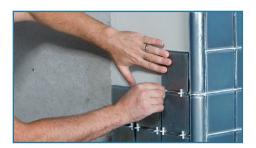
**Step 6** Press the tile into the fresh setting bed using, firm even pressure. Remove excess setting material from the edges and space a minimum of 1/8" between tiles and all abutting surfaces.
