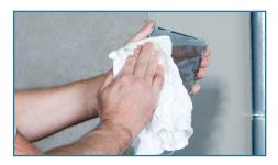
**Step 4** Thoroughly clean the back of each tile using a clean, dry cloth. Never wet the tile prior to setting.
