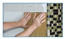
**Step 4** Apply mosaic sheets to the thin-set setting bed, paper side towards you, with light, even pressure. Periodically, check thin-set for skinning (slight drying). If skinning occurs, remove thin-set and reapply.
