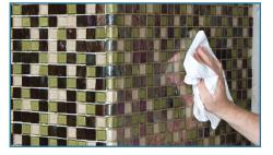
**Step 12** For final removal of grout haze, polish with a clean, soft cloth.
