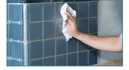
**Step 9** For final removal of grout haze, polish with a clean, soft cloth.
