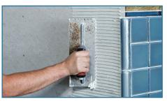
**Step 2** To establish the proper depth of the setting bed, use a 1/4"x1/4" square-notch trowel to apply additional thin-set and comb full notches in one direction.
