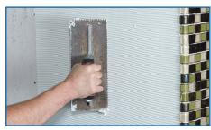
**Step 2** To establish the proper depth of the setting bed, use a 3/16"x1/4" v-notch trowel to apply additional thin-set and comb full notches in one direction.
