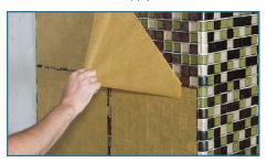
**Step 7** Peel the paper from the tile starting at the corner. Removing the paper while the setting material is still fresh allows for individual tile adjustment and re-inspection of color consistency.
