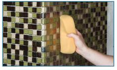
**Step 11** Allow grout to set-up (firm) and smooth finish with a damp sponge. After approximately 2 hours remove grout haze with a lightly damp sponge.
