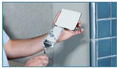
**Step 5** Back-butter each tile using additional thin-set. Prior to setting translucent tile, check the face to verify 100% coverage has been achieved.
