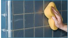
**Step 8** Allow grout to set-up (firm) and smooth finish with a damp sponge. After approximately 2 hours remove grout haze with a lightly damp sponge.
