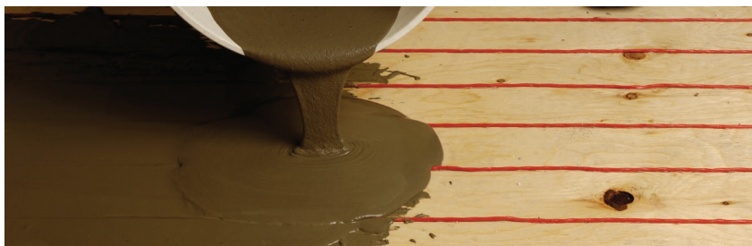
FIGURE 2.42: Self-leveling compound method
