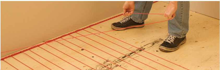
FIGURE 2.27: Install the heating cable
