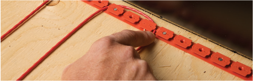
FIGURE 2.26: Install the heating cable
