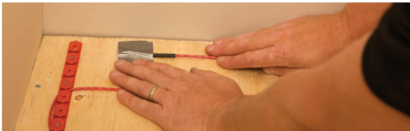
FIGURE 2.28: Secure the end seal
