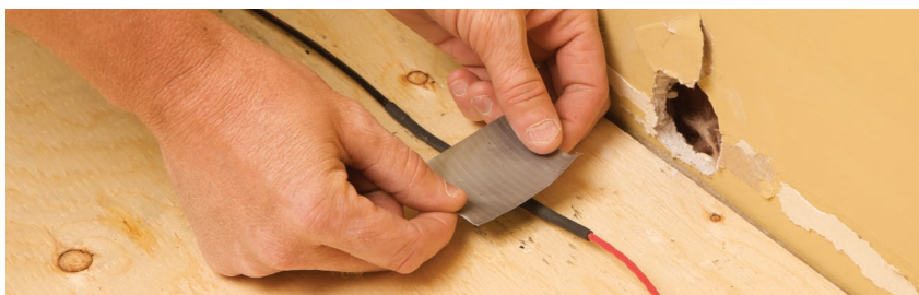
FIGURE 2.23: Secure the cold lead to the subfloor
