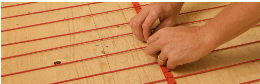
FIGURE 2.29: Install stabilizing guides
