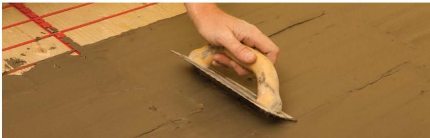
FIGURE 2.52: Thinset mortar method
