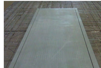
FIGURE 8 Saw kerfs for rodding.
