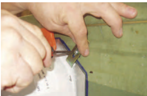
FIGURE 9 Undermount sink mounted with mechanical anchors.
