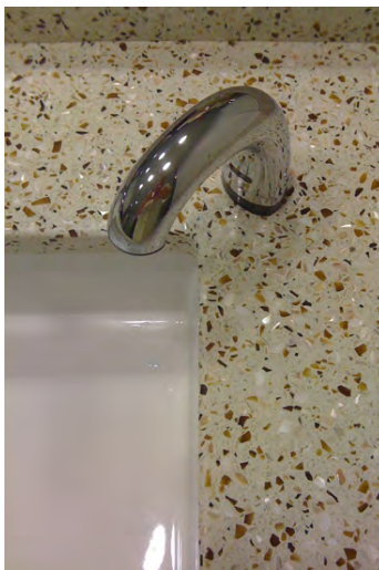
FIGURE 11 Soap dispenser should drip directly into sink bowl.
